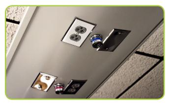
Data, communications and electrical services are delivered via two rows of junction boxes
