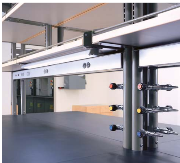
Under-shelf lighting, power and data bars, and needle-point service fixtures are designed to be within arms reach, above an obstruction-free work surface.
